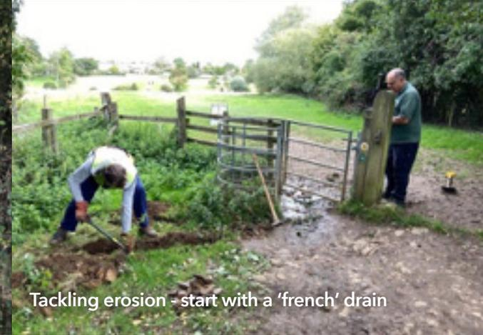
Tackling erosion - start with a 'french' drain
