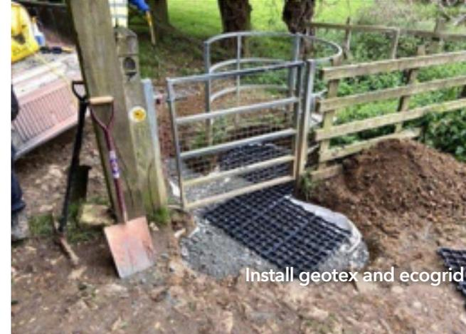
Install geotext and ecogrid
